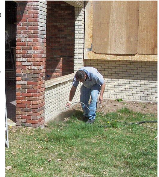
use on masonry. They have perm ratings of 9 or 10. A high perm factor indicates a paint with a high capacity to transmit water vapor.
