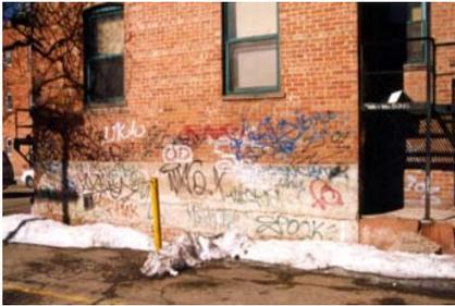
All types of cleaning are hard on masonry walls. Cleaning should only be attempted if the layer of dirt is actually harming the wall. Acid rain trapped at the face of the wall by encrusted dirt can eat away at the face of the brick. If cleaning is necessary, do several tests to determine which cleaning procedure and solution will be most effective.
